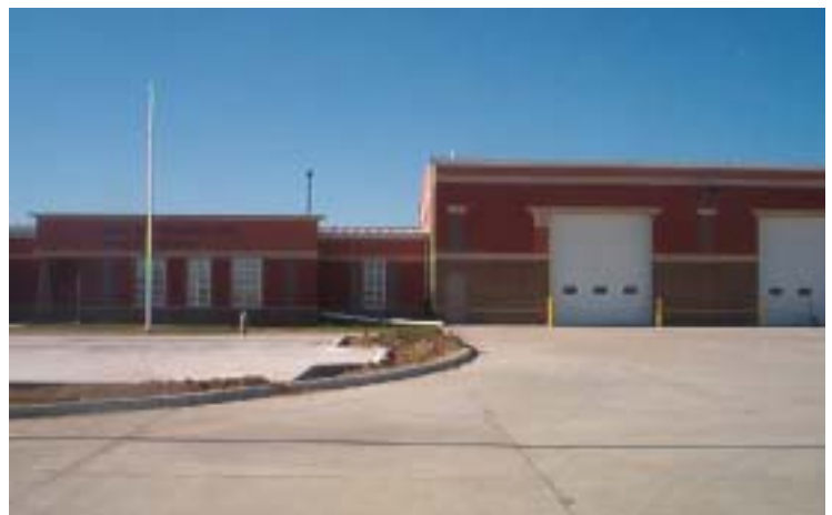
Norfolk Maintenance Facility Exterior, Norfolk, Nebraska
